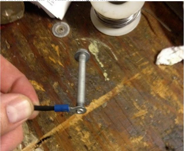
Since it was a little big, I could have used a drill to open up the hole (which is a little tricky), or what I ended up doing which was cutting the end of the loop to make it split, allowing the bolt to pass through it. I could have avoided this if I'd had an open-ended/forked solderless terminal instead of a loop, but hind-sight is 20/20.
